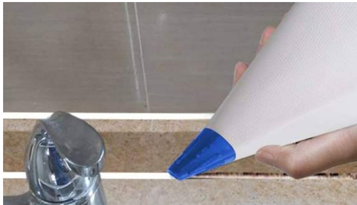
Grout Installation with Grout Bag
