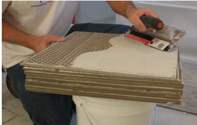
Back Buttering of Paver
